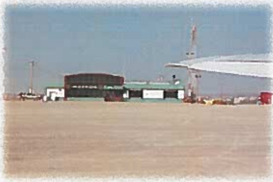
FIGURE 21 APPROACH AT THE AIRPORT
